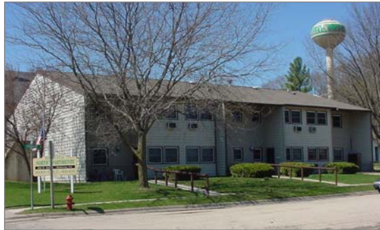
EIRHA Apartments, N Fourth St. (Source: ECIA)
