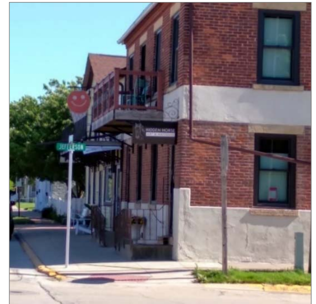
Upper story housing, N Riverview St. (Source: ECIA)
